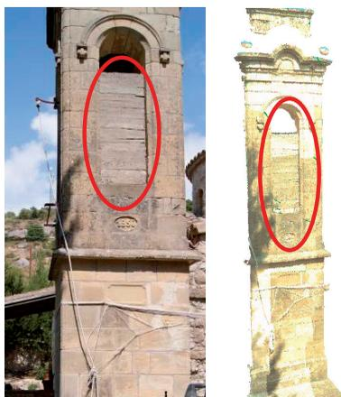
Figure 16: Documentation of anthropogenic change of the bell tower at the church of Saint Kirikos and Ioulitis. In circle the recent intervention in the church (photo in the left / 3D laser scan model in the right)
