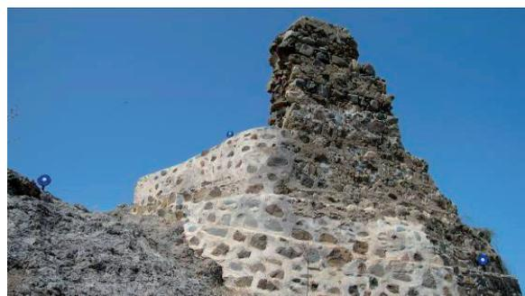
Figure 5: The north-eastern side of the edifice. Three of the special targets used for scanning this side of the monument are visible in the above image
